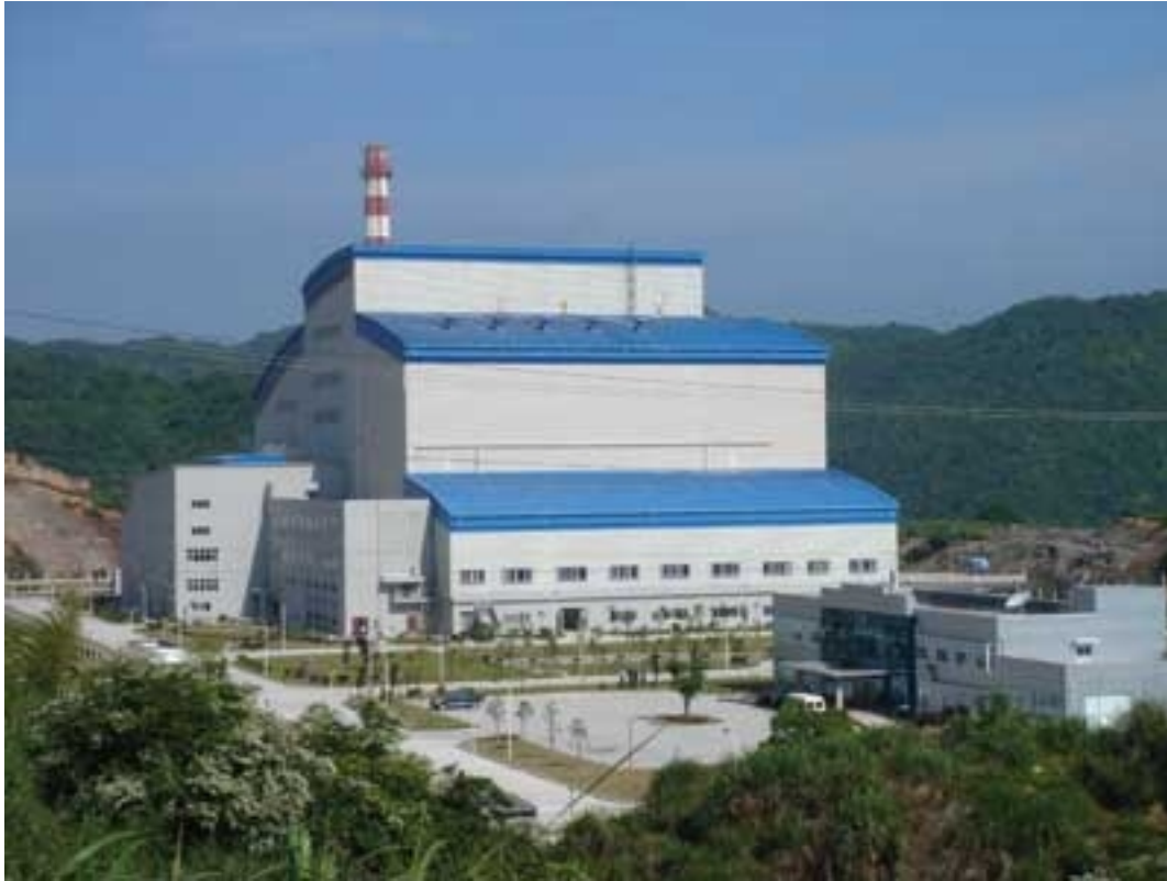
Fuzhou Hongmiaoling EfW plant
